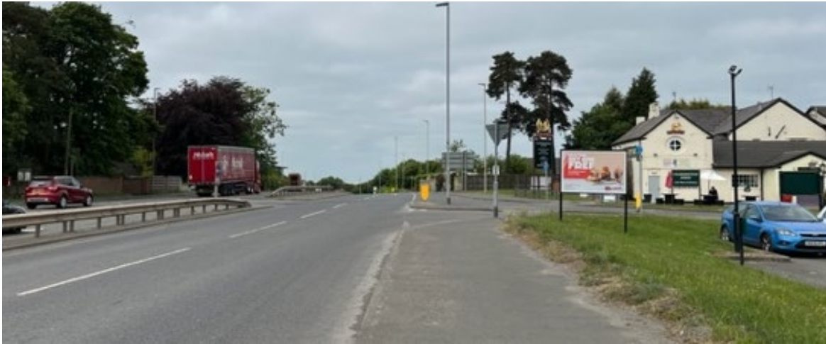
Photograph of site access looking westwards along Beveridge Lane:
